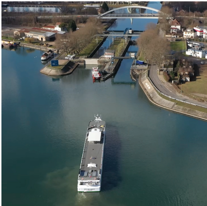
Figure 3. Automatic entering a waterway lock with MS Victor Hugo
