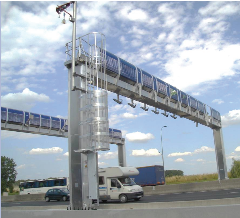
Figure 12 Sanef gantry for initial deployment of probes
